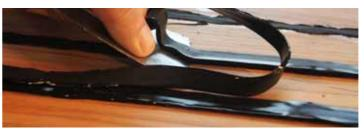
Allow the rubber to cross-link for at least 48 hours (more time is needed if temperatures are low) before trimming off excess sealant.
