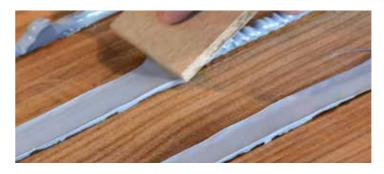
Immediately after application, run a flexible squeegee over the seam at a 30-degree angle. Apply enough pressure so that the rubber penetrates the bottom of the seam, but leave an excess layer of rubber.
