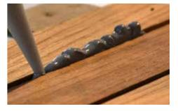
Make sure the rubber goes all the way to the bottom of the seam, allowing the rubber to slide upward until it reaches the top of the seam. Avoid starts and stops or changes in direction that can trap air.
